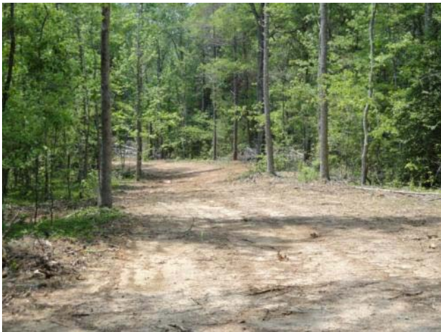
Newly graded access road
