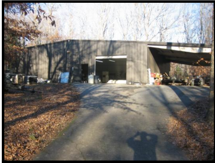
Large workshop and equipment shed
